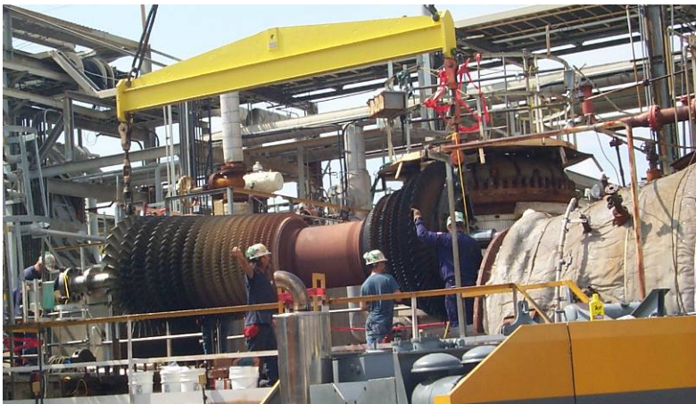
On-Site Major Overhaul of a Gas Turbine
